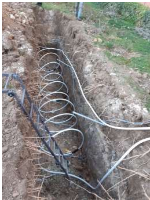
FIG. 1. VIEW OF THE GHE BURIED IN 3 M DEPTH
