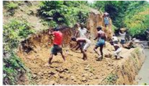
Figure 8 Hill cutting for road expansion
