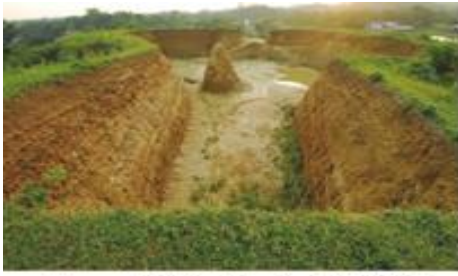
Figure 7 Hill cutting for brick field
