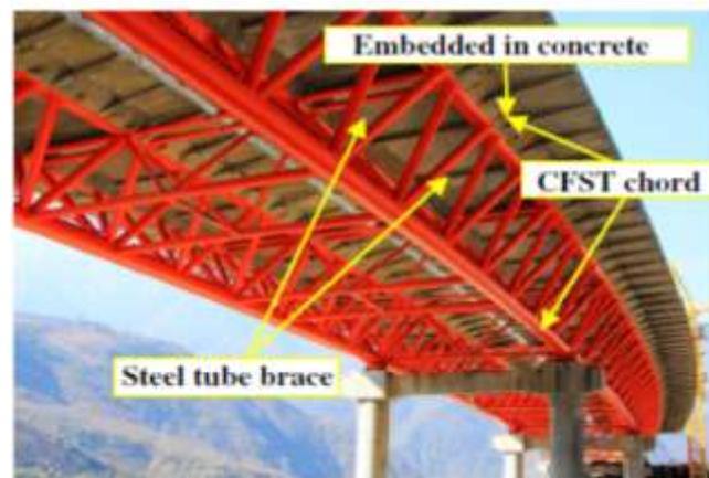
**Fig. 1** The Ganhaizi Bridge in China uses CFST trusses
