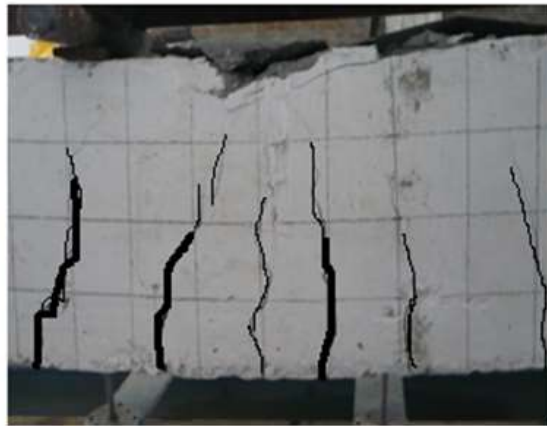
b) Bamboo Straps with binding wire winded beam
