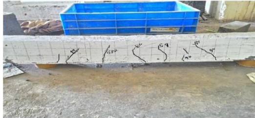
Fig. 8(b): Crack pattern for GGBS and BA
