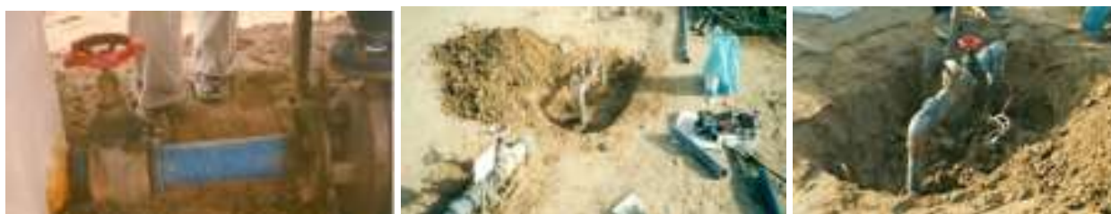
Figure 2. Irrigation systems networks maintenance.
