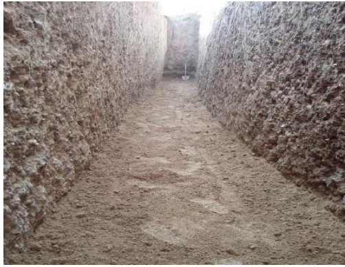
Figure .4: trench ditch.
