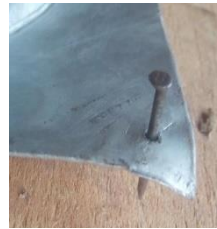
Figure 29: Nails for corners of metal to wood
