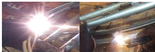
Figure 40: Welding of galvanized pipe joint
