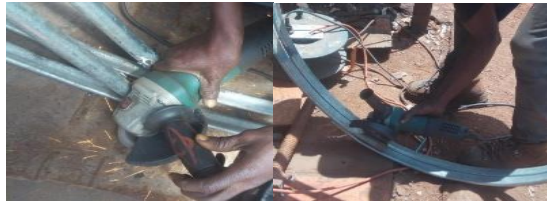
Figure 41: Grinding off bumps on joints
