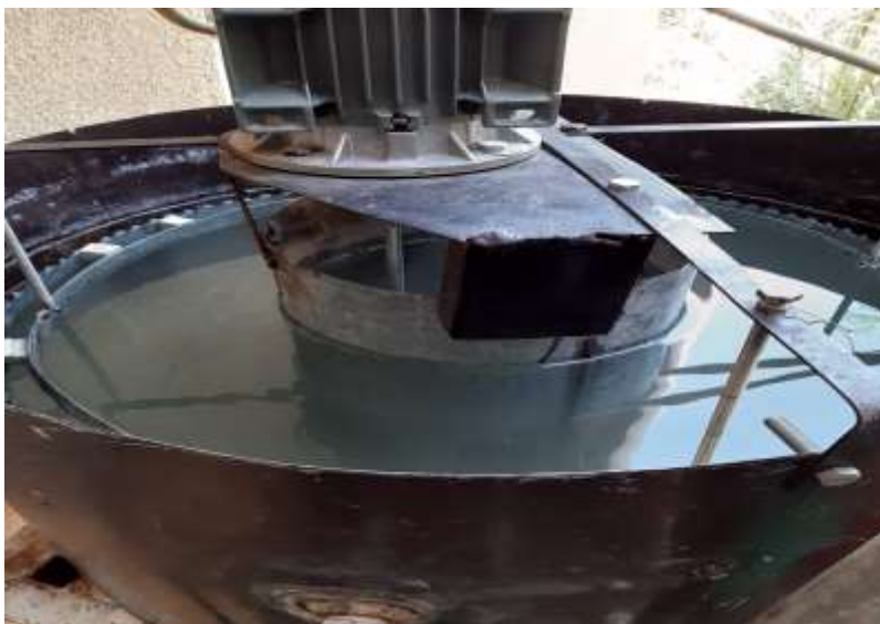
Figure 1. Flash Mixing Tank
