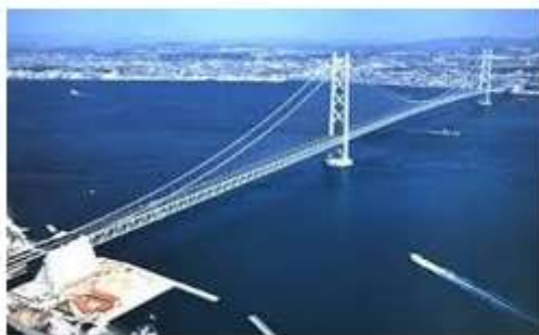
Figure 1. Akashi Kaikyo Bridge, Japan
