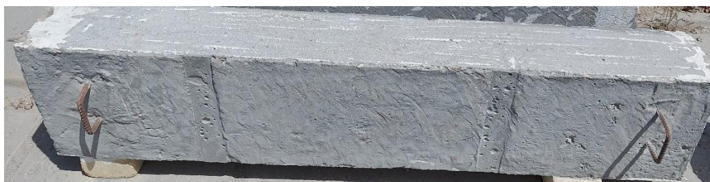
Figure (9): Cleaning surface of concrete and chamfered corners
