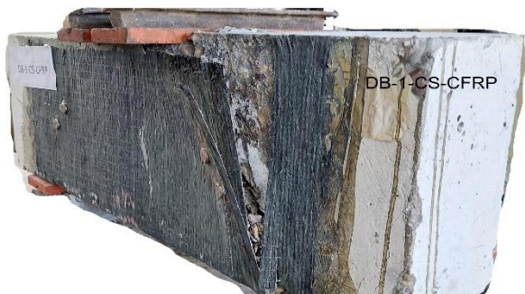
Figure (9): Failure mode for Rehabilitated Deep Beam with (a/d=1) failed in shear - DB-1-CS-CFRP
