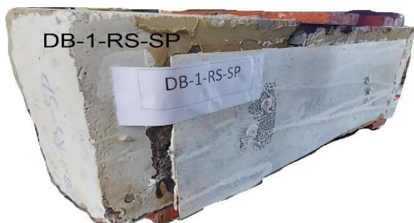
Figure (21): Failure mode for Rehabilitated Deep Beam with ( a/d=1 ) fail in shear - DB-1-RS-SP
