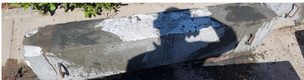
Fig (8). Repaired beams with cementitious grout
