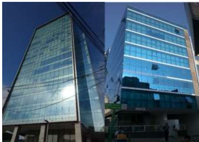
Figure 2. Leuro and Cantuarias Buildings in Miraflores
