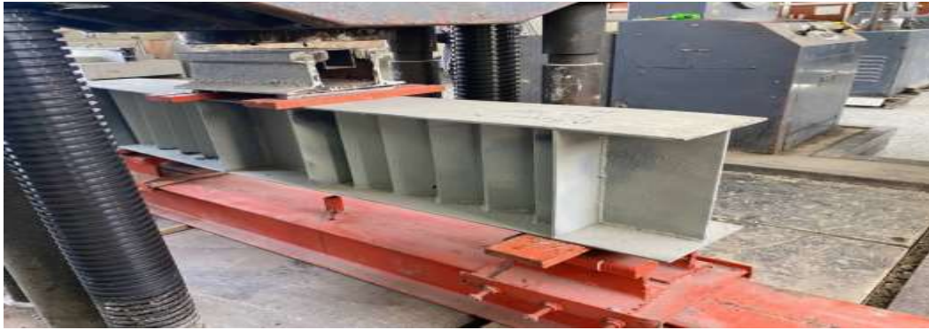
Figure 10. Preparation of Plate Girder.
