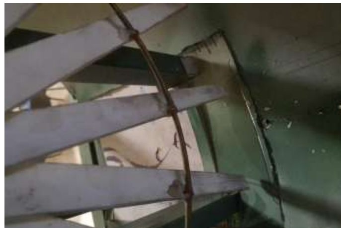
Figure (12) Blade failure in wind turbine at adhesive joint.
