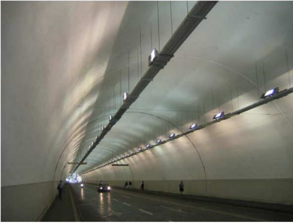
Figure 4. Application of photocatalytic coating to the internal surface of a tunnel
