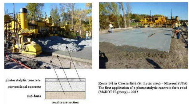
Figure 3. Two-lift technology for paving
