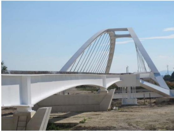
Figure 1 - Newly built bridge with concrete piles made using photocatalytic cement
