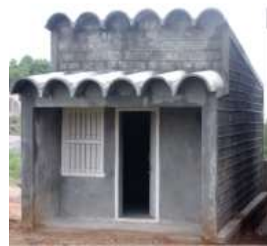
Figure 8 Example of Ferro cement Channel Construction
