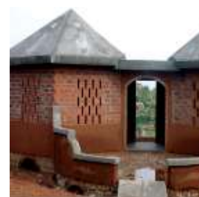
Figure 5 Rat Trap Bond Brick Wall
