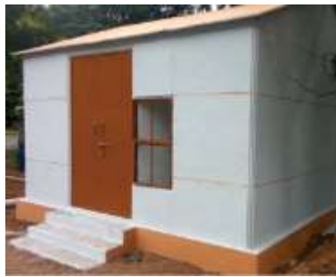
Figure 10 example of pre-fabricated steel house
