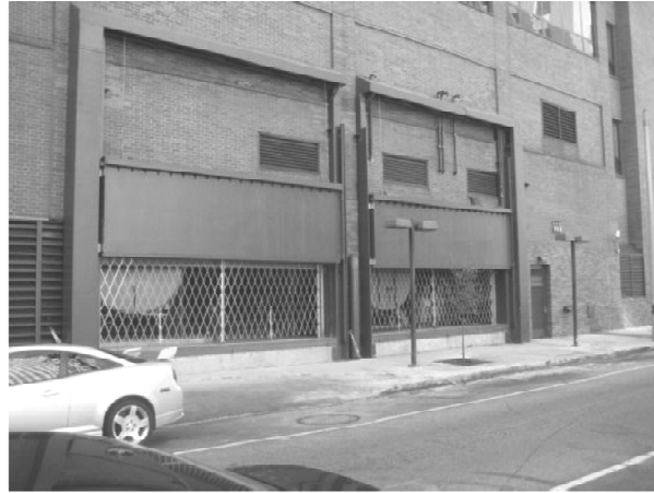
Figure 7: Vertical Guillotine Doors Prior to Flood Test
