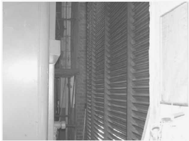
Figure 6: Louvers That Extended Below the Flood Level
