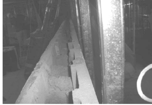
New 6 ft. tall CMU Walls with Grout Infill
