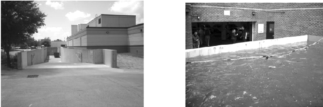
Figure 2: Passive Flood Door Before and After Activation
