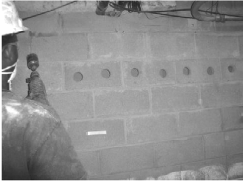
Drilling and Pouring Concrete Grout for Wall Strengthening
