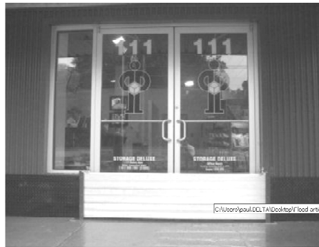
Figure 3: Simple Drop in Slat Door for Low Levels of Water
