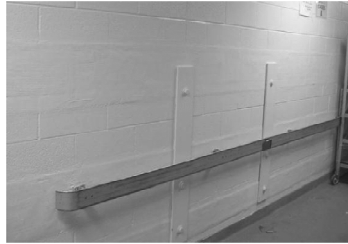
Completed Wall Strengthened and Waterproofed
