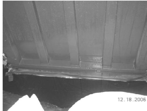
Flood Door with Six Ft of Water and No Leaks at the Door or Walls
