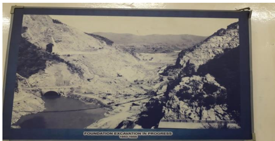
Figure – 4 Foundation work at the site
