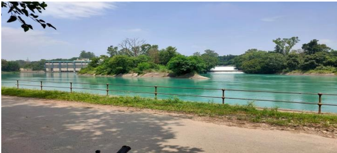
Figure – 10 Ganguwal Power House
