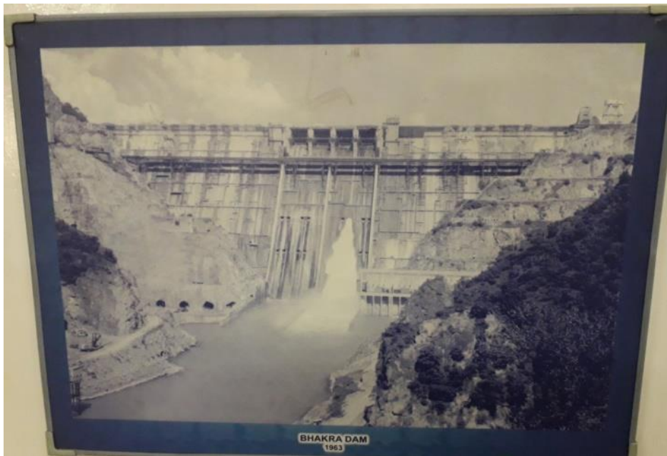
Figure – 6 final work at the site
