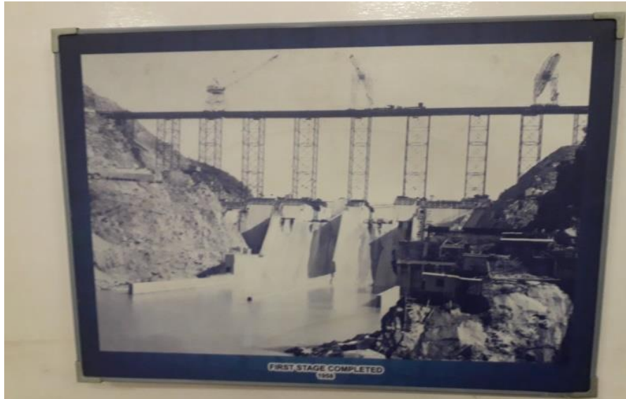
Figure – 5 Laying of Slab for the Dam
