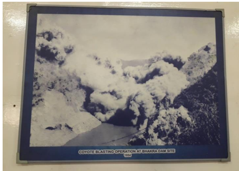
Figure – 3 Blasting at the site of Bhakra Dam
