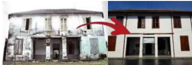
Figure 5. Changes in Window Forms on Building Facades (Doc. Author, 2020)
