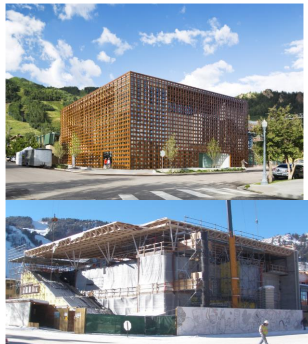
Figure (17) shows the Aspen Museum of Art building and its affiliation with the surrounding nature. It also shows the use of wood treated with nanotechnology in making the ceiling of the last floor of the building. 21
