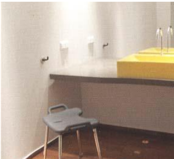
Figure (30) the use of easy-to-clean, anti-scratch and anti-steam surfaces in the bathrooms of patient rooms in order to save maintenance costs and not to condense water vapor on the mirrors. 5
