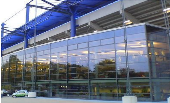
Figure (5) shows the glass facade of the building from the outside and the inside, which works with self-cleaning nanotechnology, as well as noise isolation and protection from sunlight. 11
