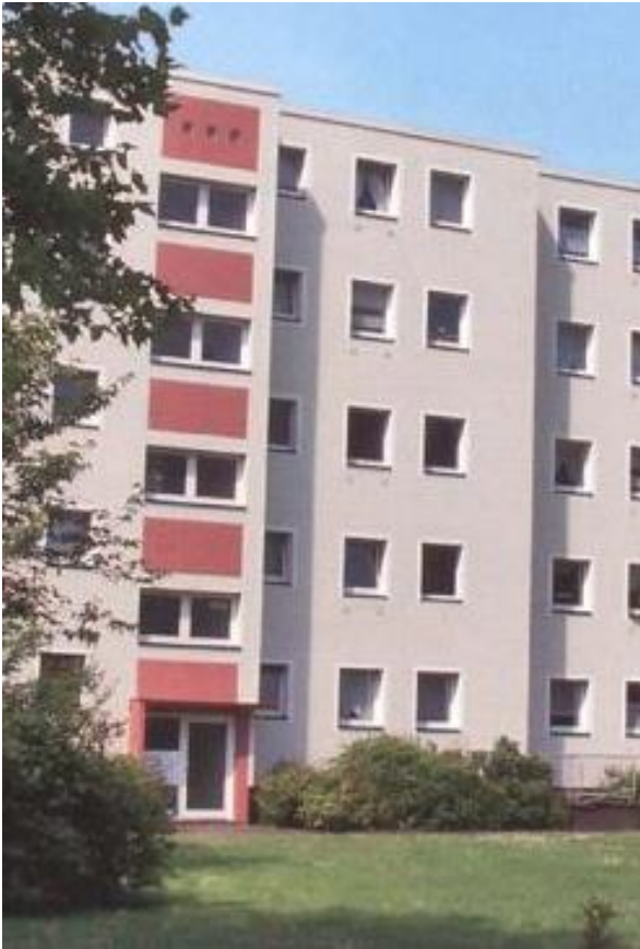
Figure (13) shows the building after being treated with an anti-bacterial nano coating. 14
