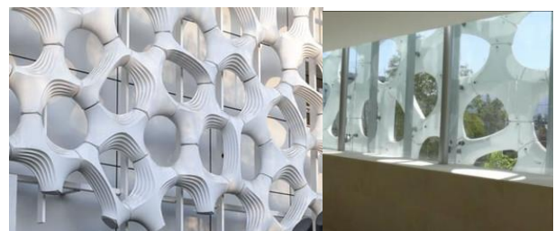
Figure (26) shows the facades of the hospital in which brick panels are used with air purification technology and the reduction of pollutants, which also serves as a canopy for the facade of the hospital. 34
