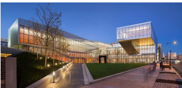
Figure (23) shows the building's glass facades that are self-cleaning, anti-bacterial, anti-scratch, and have high thermal and acoustic insulation (nanogel). 30
