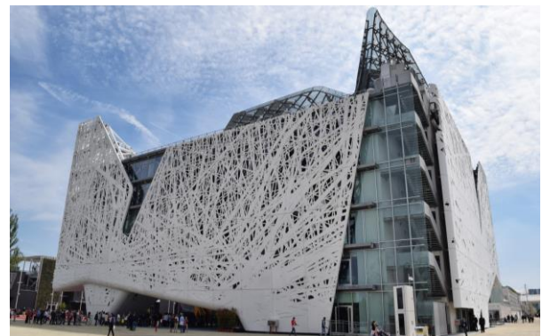
Figure (7) shows the building of Expo Milano 2015 - The Italy Pavilion, which consisted of white, irregularly shaped façades, punctuated with openings, and the façades were made of a mixture of cement and titanium dioxide. 13
